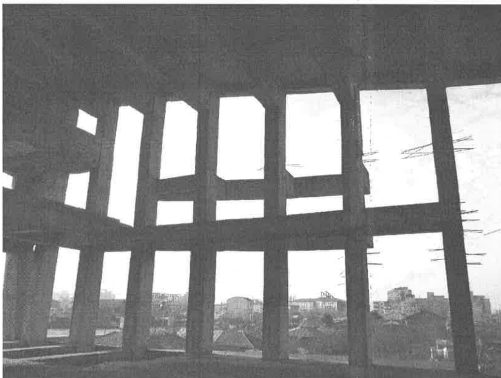
DETALIU INTERIOR CORP A – PERETE VEST
